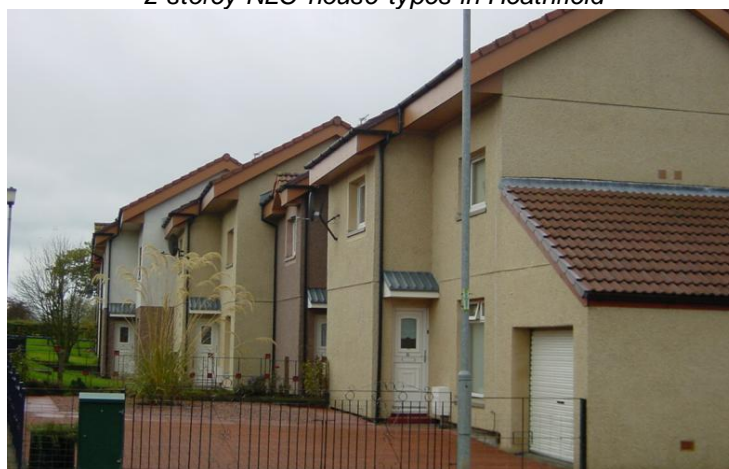
2 storey NLC house types in Heathfield
