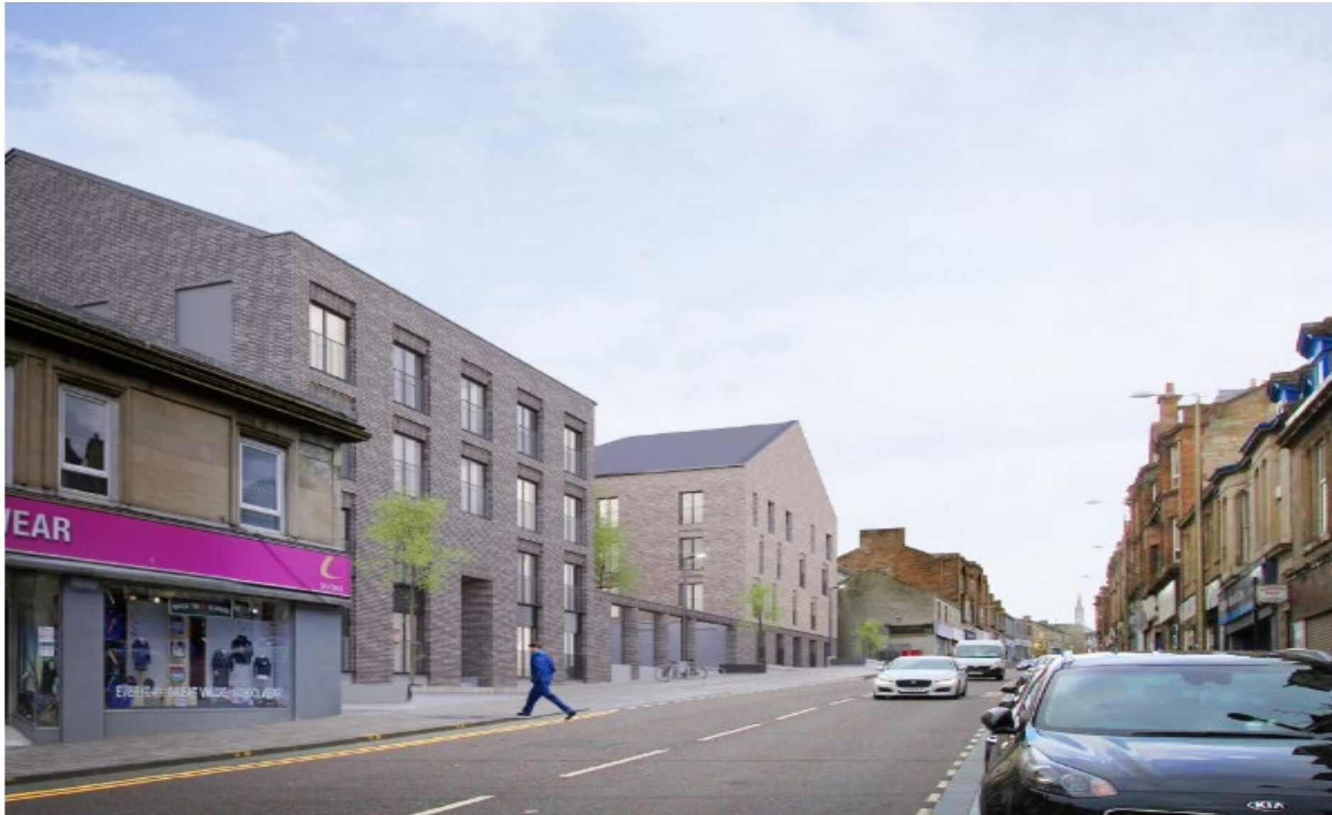
Exemplar urban infill residential flattened accommodation, Main St, Wishaw (former Anvil Block)
