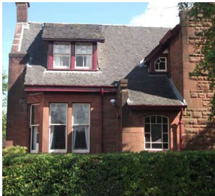
Traditional details and materials enhance the character and help ensure value is retained.
