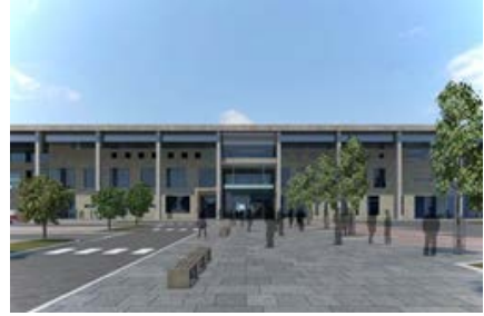
Greenfaulds High School
