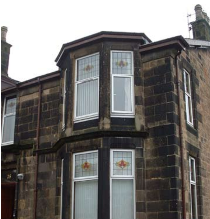
In some instances windows are replaced with UPVC without consent, which would be a breach of regulations and may cause difficulties with a future sale.
